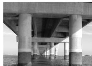
Surface encapsulation with glass fiber (APE)
