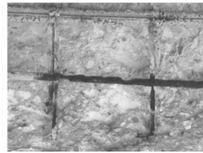
Localized Corrosion
