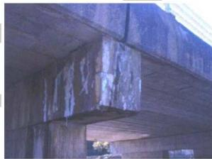
Figure 3 – Cracking, leaching and staining on the crossheads
