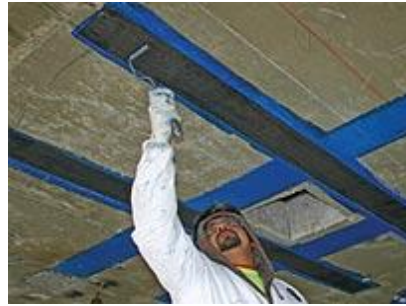
Fig 4. Application of FRP strips
