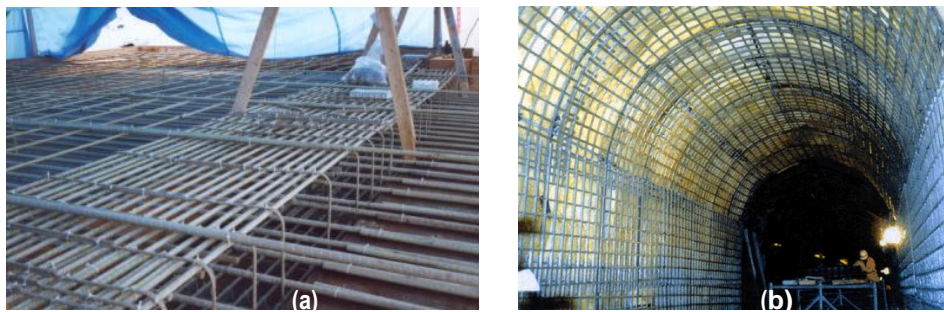
Fig. 10. Application of FRP as concrete reinforcement in new structures: (a) bridge deck; (b) underground tunnel
