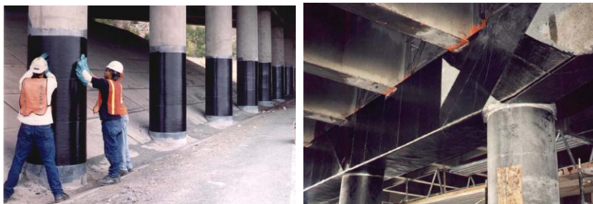
Fig 5. Seismic retrofitting of a bridge with FRP composites
