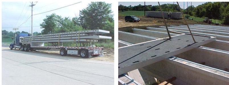
Fig 7. Example of a FRP bridge deck system
