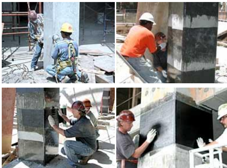
Fig 3. Wet lay-up of FRP sheets
