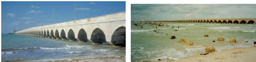
Fig. 10. Pier of Progreso de Castro, Yucatán, Mexico. Structure built from 1937 to 1941 with stainless steel reinforcement (adapted from [16]).
