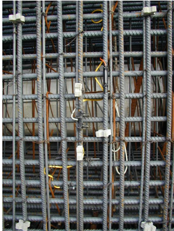
Fig. 9. Sensors before concreting.
