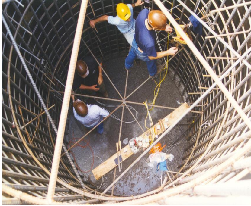
Fig. 6. Instrumentation of pier.
