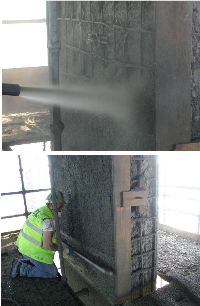
Fig. 14. Aspects of the reposition of concrete cover after the instrumentation in a zone were all the concrete cover was removed.
