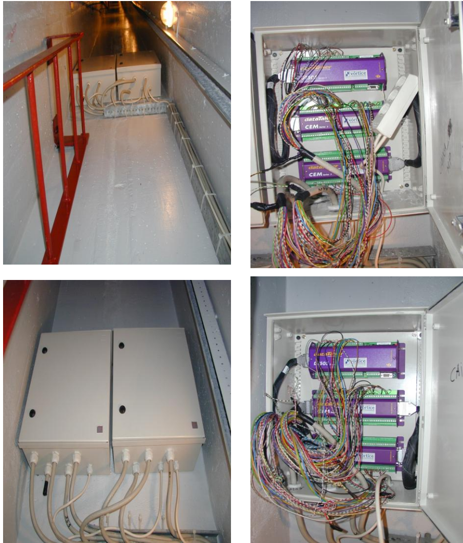
Fig. 24. Aspects of the automatic data acquisition systems installed inside the bridge.
