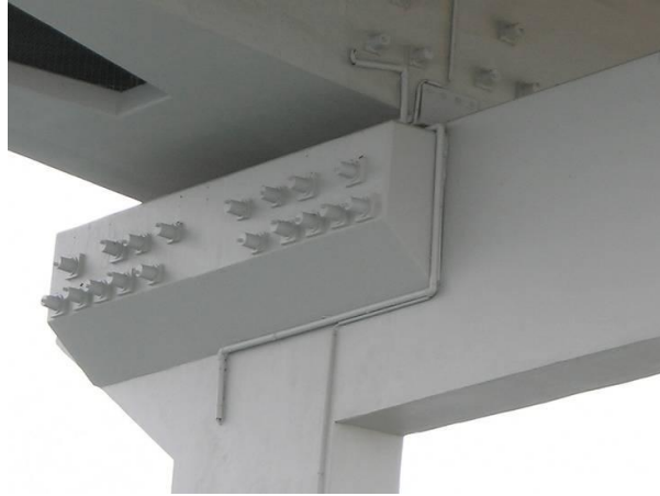
Fig.16. Cables from the sensors were conducted through external pipes to centralization boxes where the systems of data acquisition were installed.
