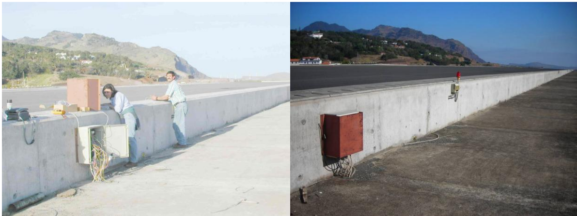
Fig. 7. Centralization box installed next to the airport runway that receives all information from sensors installed in beams and deck slab. Top – during the installation of automatic acquisition of data. Below – ten years after.
