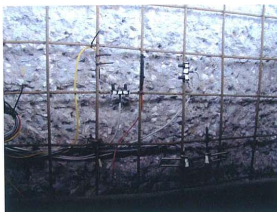
Fig. 18. Instrumentation of the pier.
