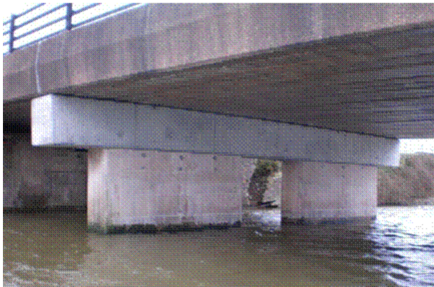
Fig. 5. Intermediate Support at Ferrycarrig Bridge
