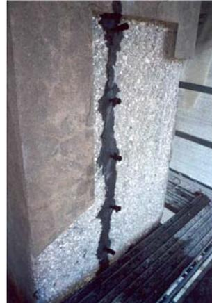
Fig.3.3 - Crack injection in columns
