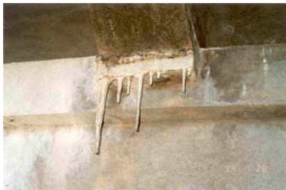
Fig.1.3. - Effects of the water penetration
