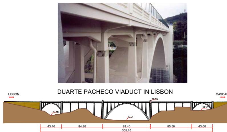
Fig. 3.1 - General dimensioning (dimensions in meters)
