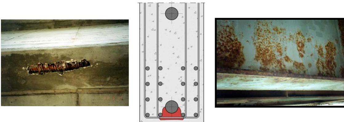
Fig 7.4 - Concrete defects in prestressed girders and corrosion in main steel beams of the cable stayed bridge
