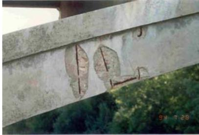
Fig 1.5 - Local corrosion
