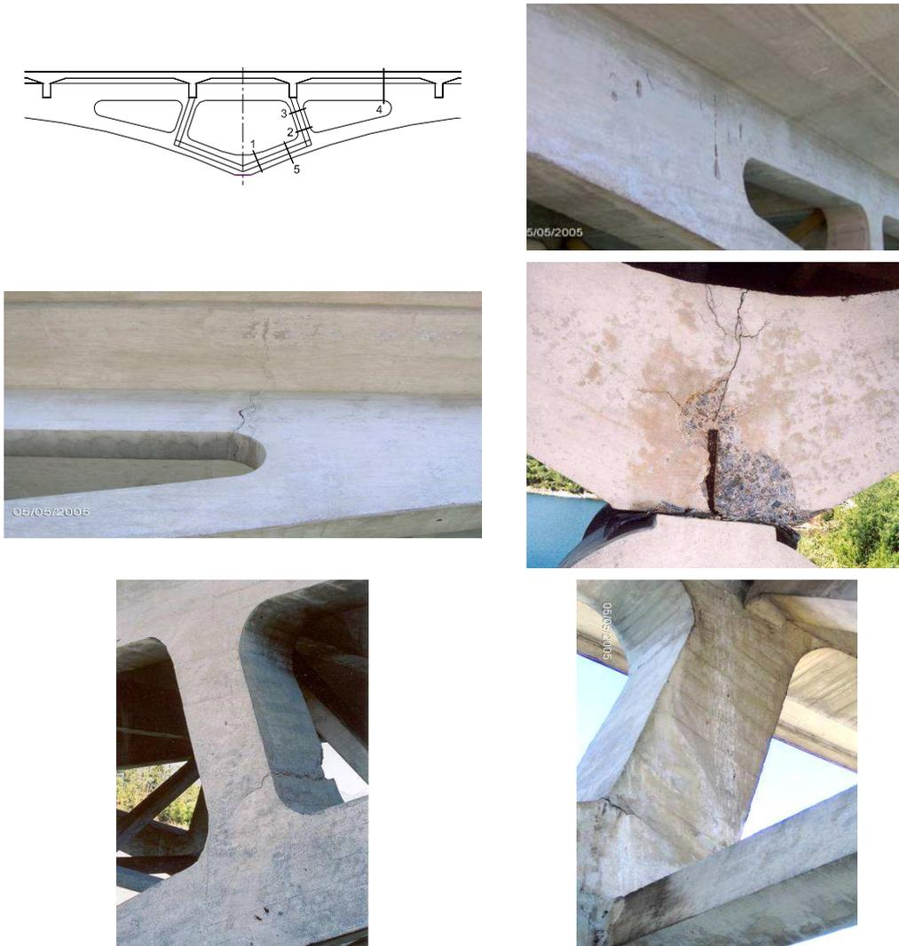
Fig 4.2 - Main structure cracking in the girder deck
