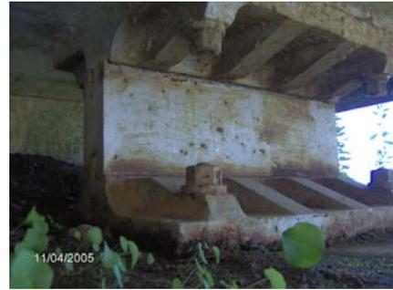
Fig 2.4 - Bearings at the abutments
