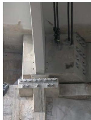
Fig. 7.7 - Details of the changes in the abutment to introduce the dampers
