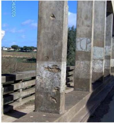
Fig 2.3 - Local reinforcement corrosion
