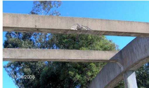
Fig 2.6 - Vehicle impact in a transverse beam
