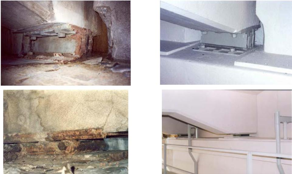
Fig 3.6 - Bearing rehabilitation and bearing replacement
