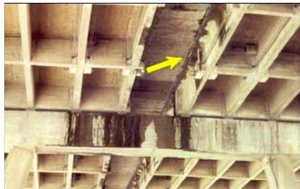
Fig 5.3 - Water penetration from the deck
