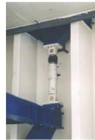
Fig. 5.6 - Details of the new supporting structure and viscous dampers
