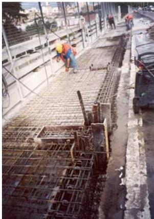
Fig 3.7 - New cantilever slab
