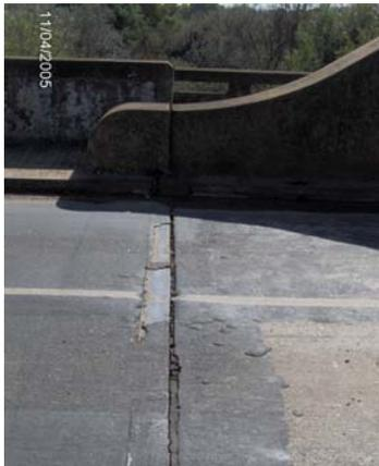
Fig 2.5 - View of the expansion joints
