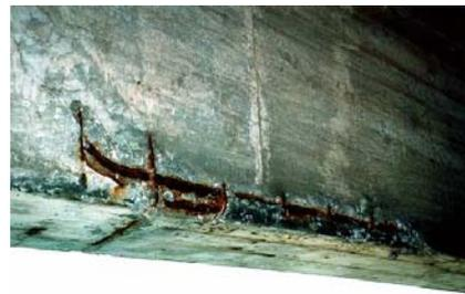
Exposed bars in construction joints and low cover regions
