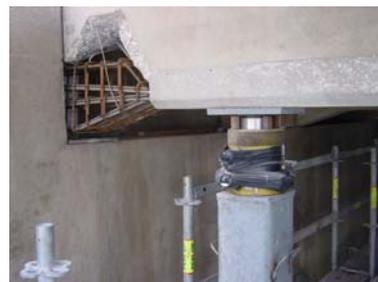
Fig 3.8 - Reconstruction of girder support region
