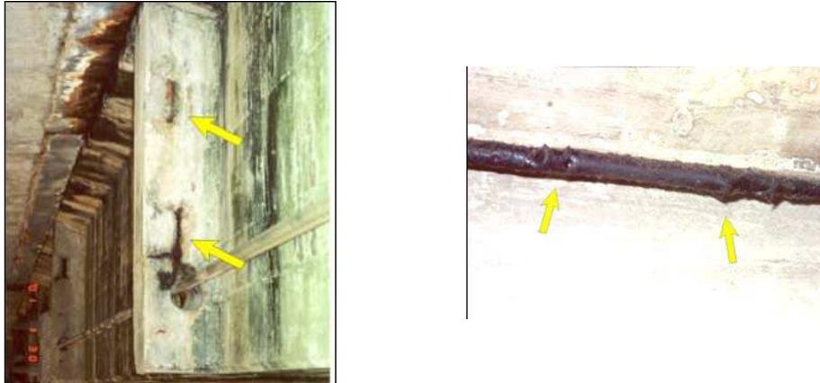
Fig. 5.4 - Damages in concrete anchorage regions and in the plastic duct of the mono-strands
