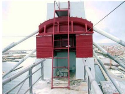
Fig. 7.6 - General rehabilitation of the saddles
