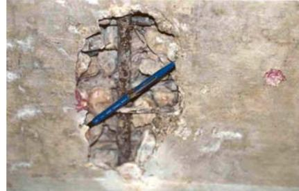
Fig 1.6 - Segregation of concrete
