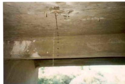
Fig. 1.4 - Water leakage from the slab
