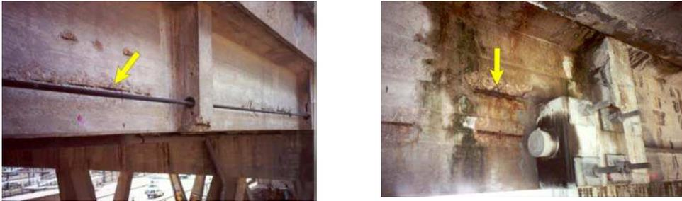
Fig 5.2 - Horizontal web reinforcement exposed due to corrosion
