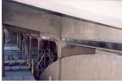
Fig 3.9 - Strengthening of lateral girders with CFRP laminates
