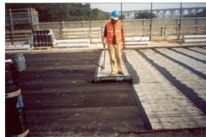
Fig. 3.5 - Deck waterproofing membrane
